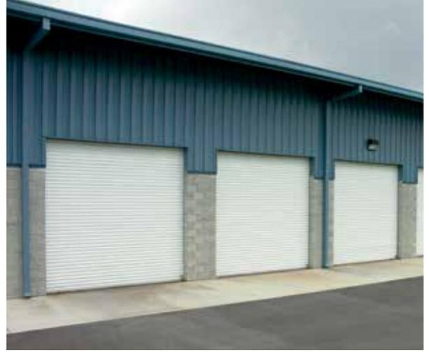
The Amarr light-duty commercial sheet door is an excellent choice for projects requiring value. The enclosed barrel assembly allows this door to fit into spaces with low headroom requirements. The Amarr 5401 and 5451 provide further value with the brackets, tensioner, gears and chain drive\* factory pre-assembled on the door saving installation time.
