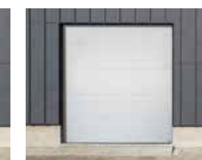
REPAIRED DOOR WITH AMARR 2747 REPLACEMENT SECTION
