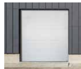
REPAIRED DOOR WITH AMARR 2747 REPLACEMENT SECTION
